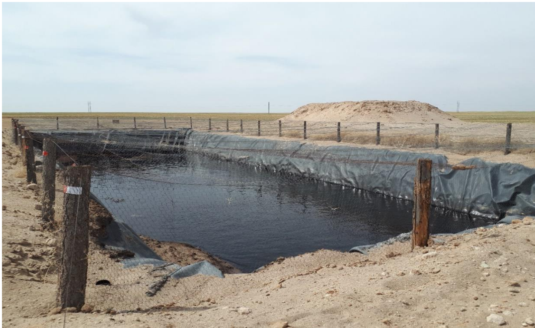
Sump being used for permanent disposal of liquid drilling waste.
