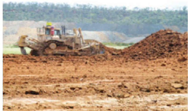
Photo 28. Stripping process the fertile soil
