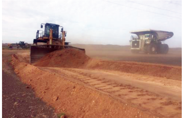
Photo 14. Stripping by dozer
