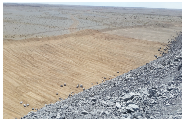
Photo 17. SGS stripped area
